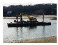
Corps of Engineers has determined that approximately 60,000 cubic yards of sediment, comprised of roughly 22.5% gravel and 76.5% sand, will be removed from the harbor inlet.
